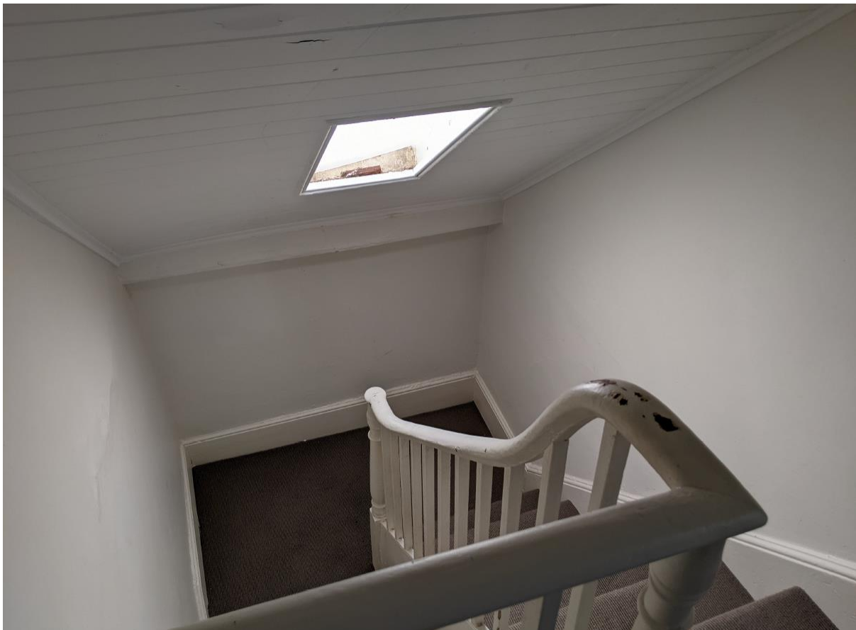
Figure 6: Existing stairs up to attic level
