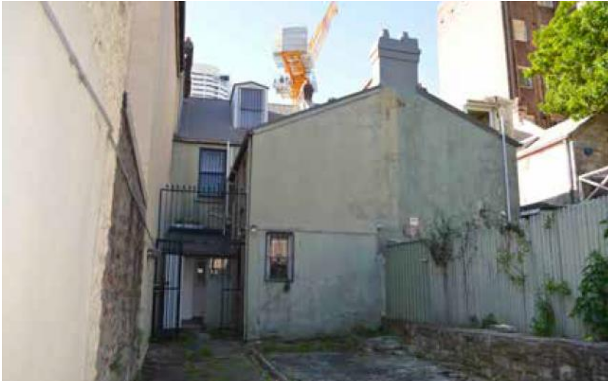
Figure 5: Existing view of the rear elevation from rear boundary (Source: Heritage Impact Statement, prepared by Zoltan Kovacs Architect and dated June 2021)
